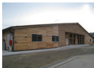
14. Watari Child Care Center (Watari, Miyagi) Disaster-stricken wood used for the external panels
