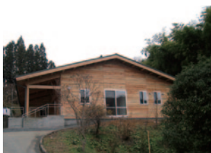
13. Ashinome Kindergarten Child-Rearing Support Center (Kesenuma, Miyagi) This center was constructed as a child-rearing support center for the area
