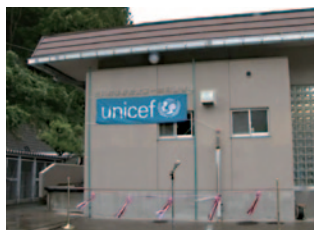
Supported repairs for the Onagawa School Lunch Preparation Center
