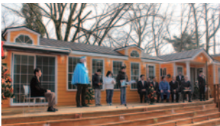
Onagawa Orange House is an after-school care facility on weekdays and a place for mothers to gather on weekends
