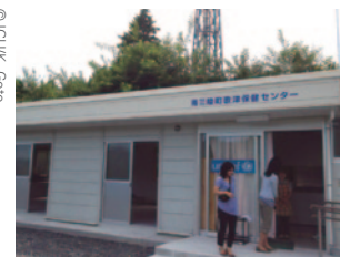
Minamisanriku Utatsu Health Center
